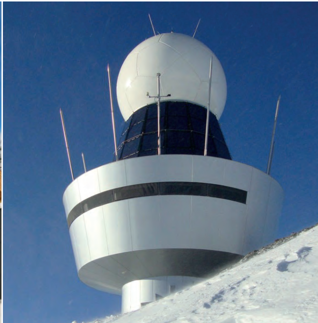
Wetterstation - weather station | Plaine de Morte | Switzerland
