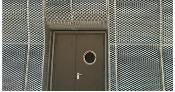
AUTOPIA / MESH CEPHE / DARA KIRMIZITOPRAK & GÖKHAN AVCIOĞLU MİMARLIK AUTOPIA / MESH FACADE
