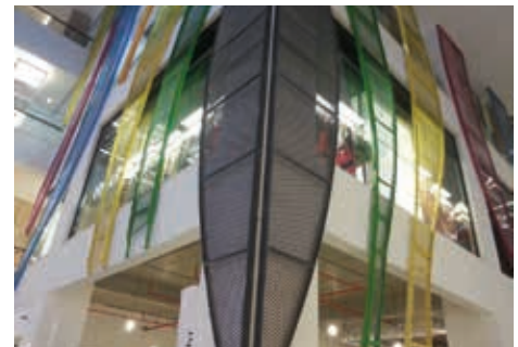
NOVADA AVM / MESH KAPLAMA NOVADA MALL / MESH CLADDING
