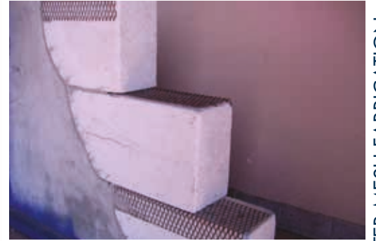
RABİS TELİ İMALATI / PLASTER MESH FABRICATION
