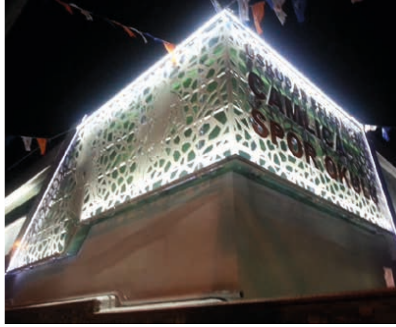
RINGS İSTANBUL / LAZER KESİM VE MESH CEPHE / HAKAN KIRAN MİMARLIK RINGS İSTANBUL / LASER CUT AND MESH FACADE
