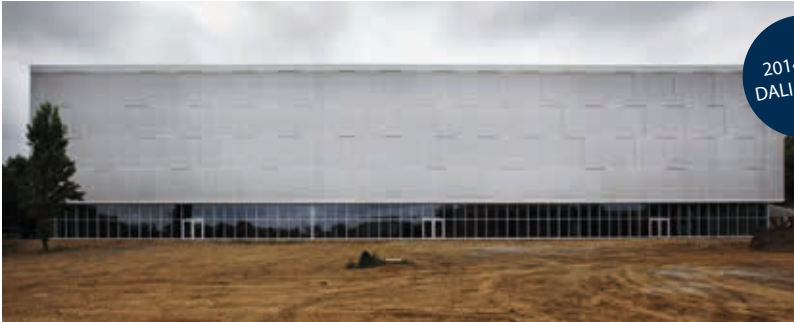
İSTANBUL TEKNİK ÜNİVERSİTESİ / UZAKTAN KUMANDA KONTROLLÜ KAYAR PERFORE CEPHE / ÖZSOY MİMARLIK İSTANBUL TECHNICAL UNIVERSITY / REMOTE CONTROLLED PERFORATED FACADE
