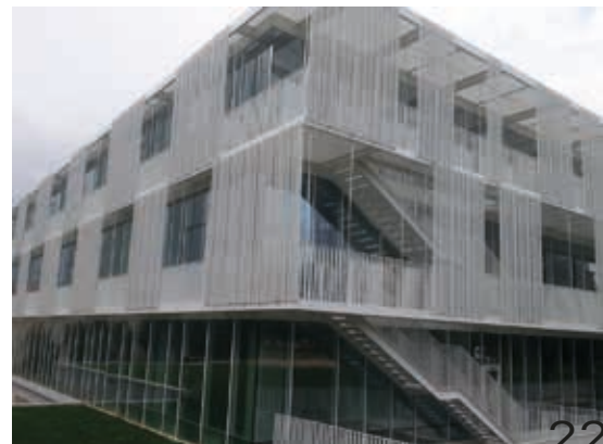
KOÇ LİSESİ / PERFORE CEPHE / DB MİMARLIK KOÇ HIGH SCHOOL / PERFORATED FACADE
