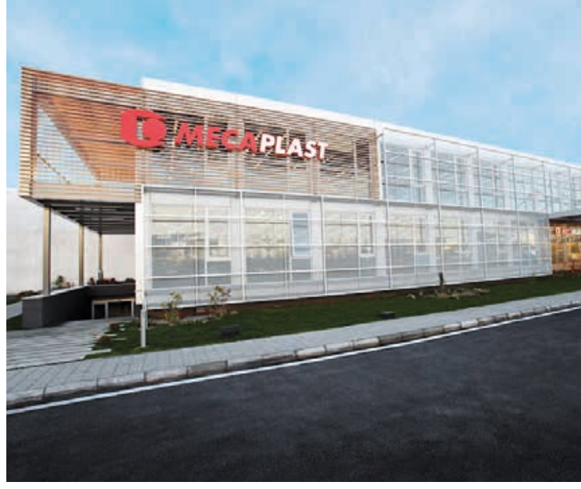
MECAPLAST AR-GE MERKEZİ / MESH CEPHE / İGLO MİMARLIK MECAPLAST R&D CENTER / MESH FAÇADE
