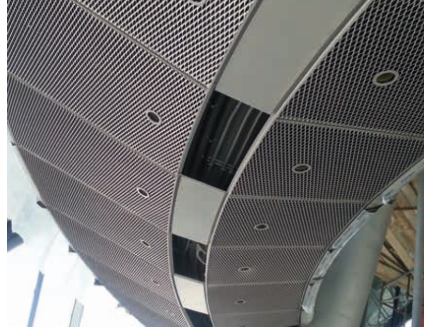
MAKKAH CLOCK ROYAL TOWER HOTEL/ MESH ASMA TAVAN MAKKAH CLOCK ROYAL TOWER HOTEL / MESH CEILING
