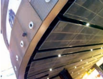
Forum Marmara / Cephe ve Tavan / Facade and Ceiling
