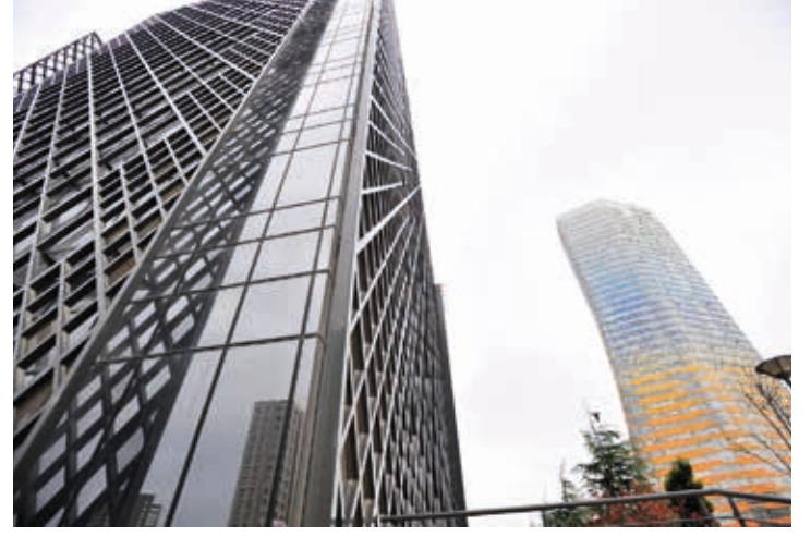
VARYAP MERIDIAN / CEPHE ANKRAJ VE HOOK / RMJM VARYAP MERIDIAN / FAÇADE ANCHORAGE AND HOOKS
