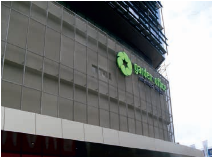
MARMARA FORUM AVM / MESH CEPHE / TABANLIOĞLU MİMARLIK MARMARA FORUM MALL / MESH FACADE
