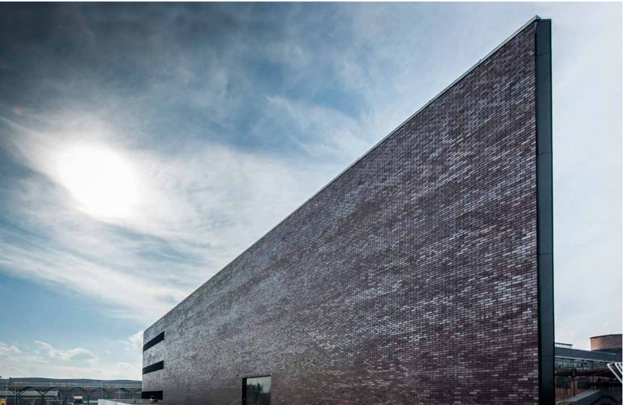
Science and Technology Centre in Ostrau (CZ) | AP ATELIER, Josef Pleskot, Prag | ADELAIDE burgund , NF
