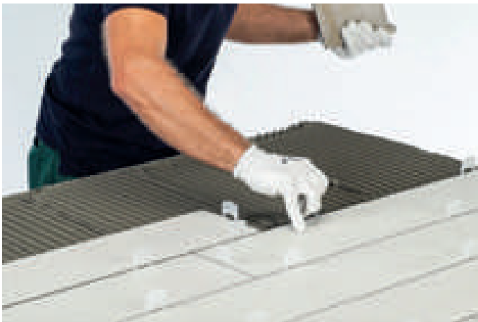
disposable clips installation
