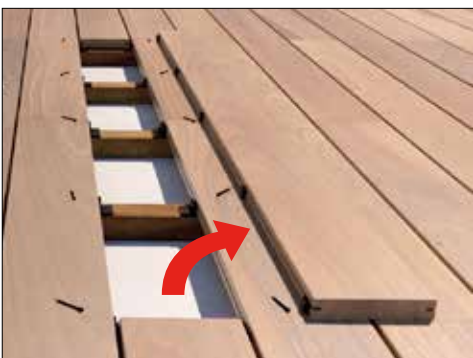
removing the board
