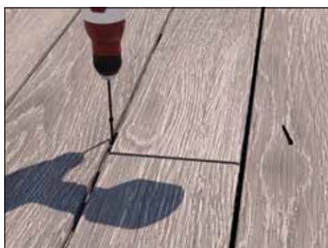
removing screws
