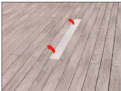
identifying boards for replacement
