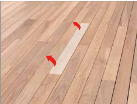
identifying boards for replacement
