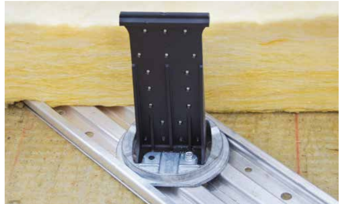
Kalzip DuoPlus on trapezoidal steel deck
